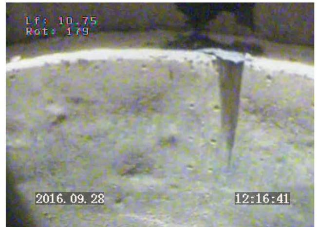
**Cuvelage en 2000mm en bon état de 11,05m à 36m.**
